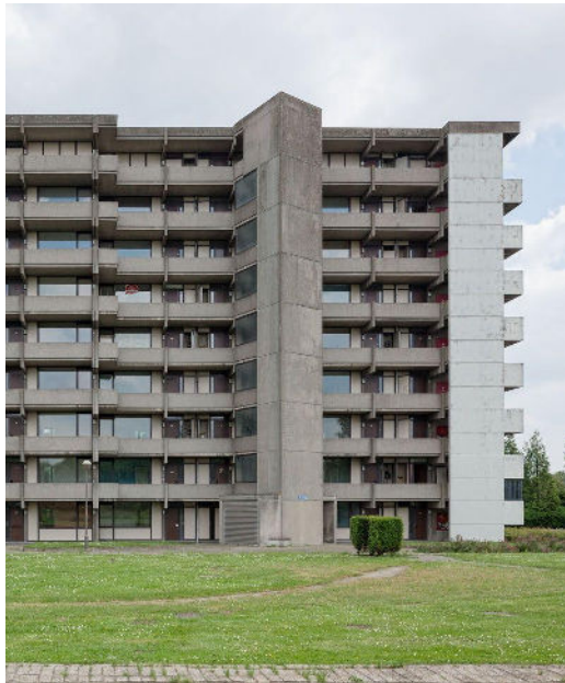
Atelier Kempe Thill - Rozemaai housing - Anvers
